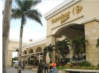
Expansion of Altos del Prado Shopping Center in Barranquilla (Colombia), with an additional 1,517 m 2 of GLA.
