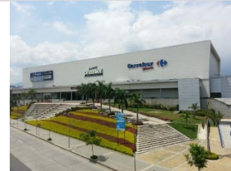
Expansion of Limonar Shopping Center in Cali (Colombia) with the addition of 2,371 m 2 of GLA.
